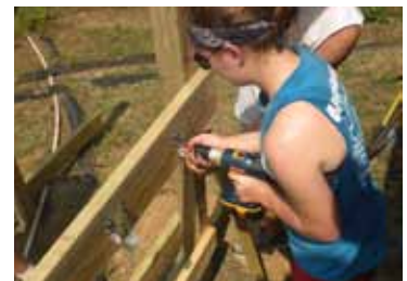
Rachel Corell uses her drilling skills to build a frame.
